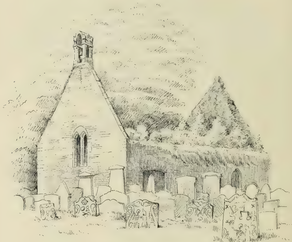
FIG. 1327.—Alloway Kirk. View from North-East.
